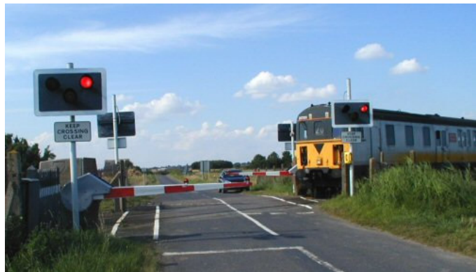
Automatic Half Barrier Level Crossing equipped with a Public Emergency Telephone System (PETS)
